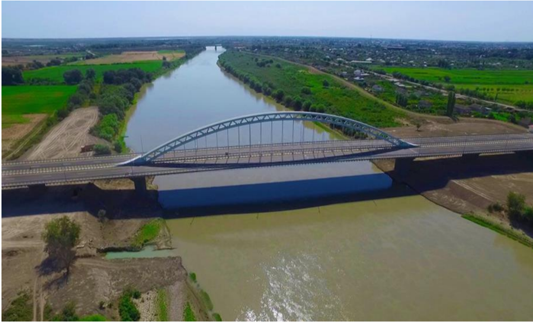
Fig. 2. Crossing roads through the bridge over the river
